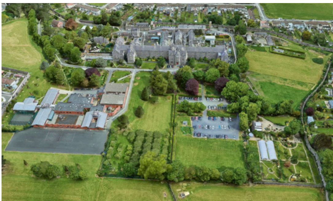
Figure 1 - Aerial photograph of site c2020
